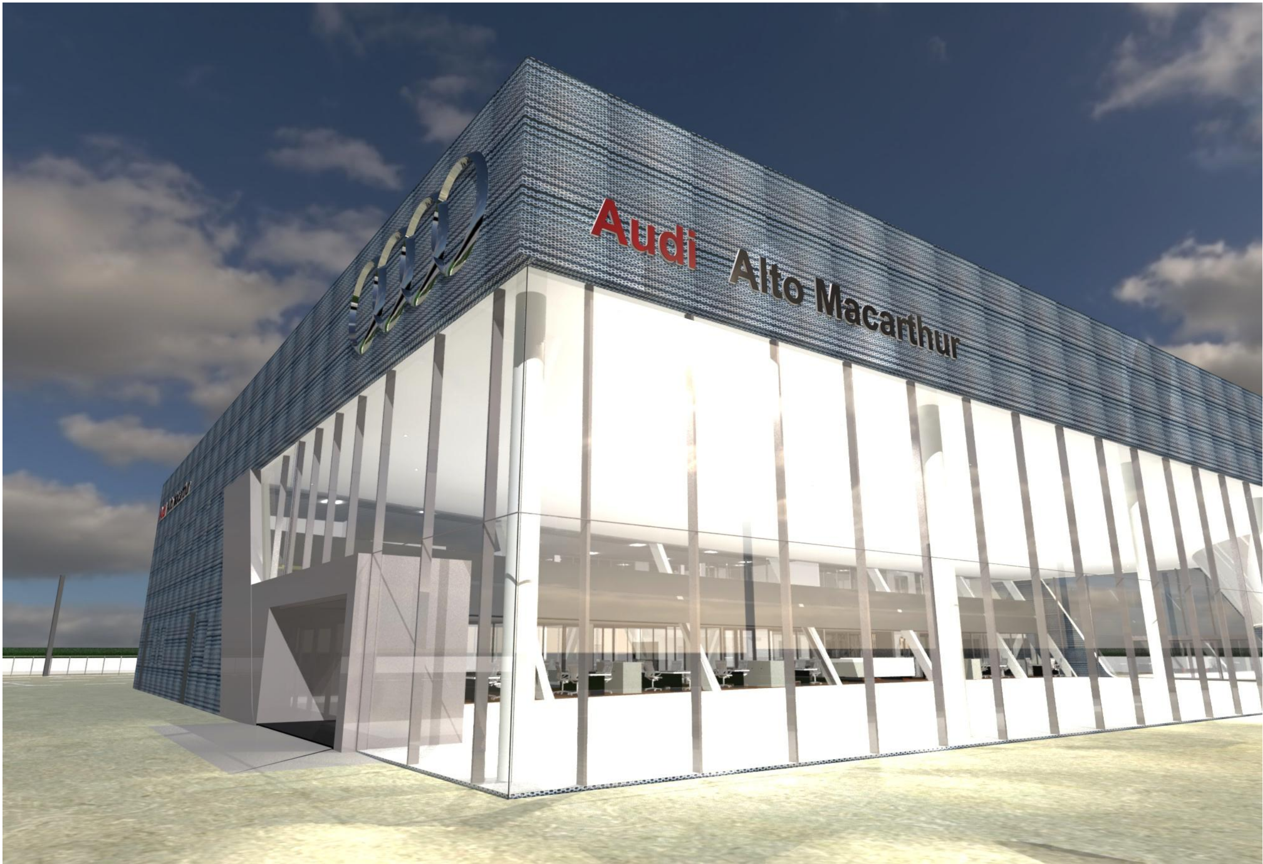
CLOSE UP VIEW OF SHOWROOM
